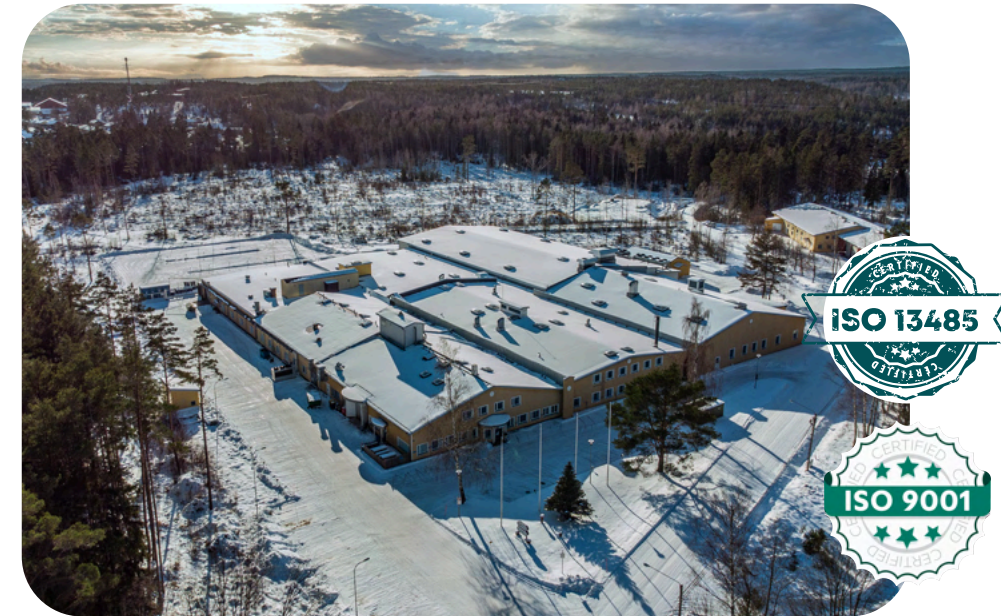
On the picture: Godby Factory / Medical segment production Åland, Finland
